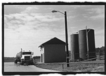
Figure 11. Ozarka's pumping station in Henderson County, Texas. Biggest Pump Wins (photograph by Mark Graham).
